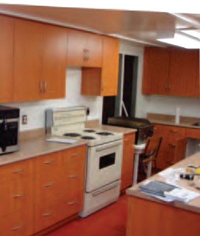
Newly refurbished cookhouse at Camp Maryglen
